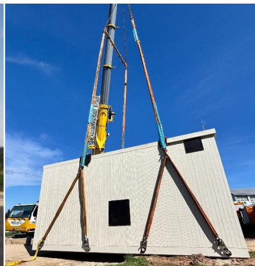
Less than 24 hours to install the modules
