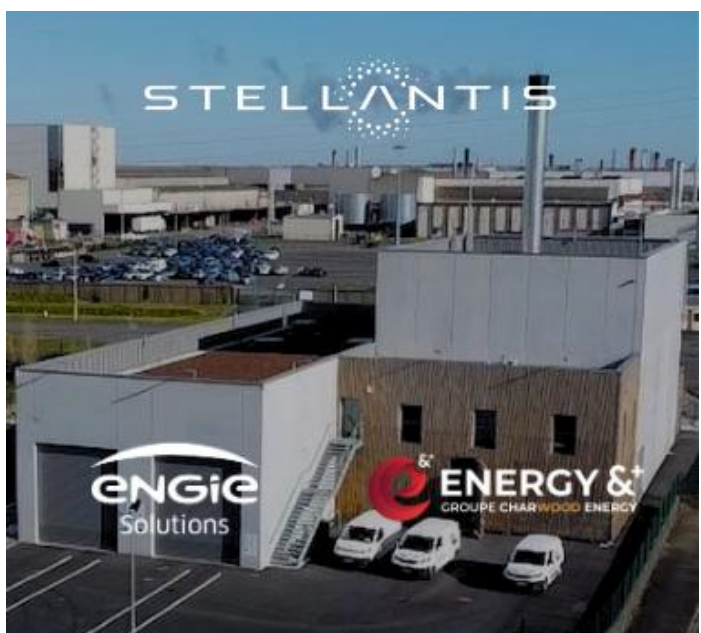
Building for the site's first biomass boiler units
